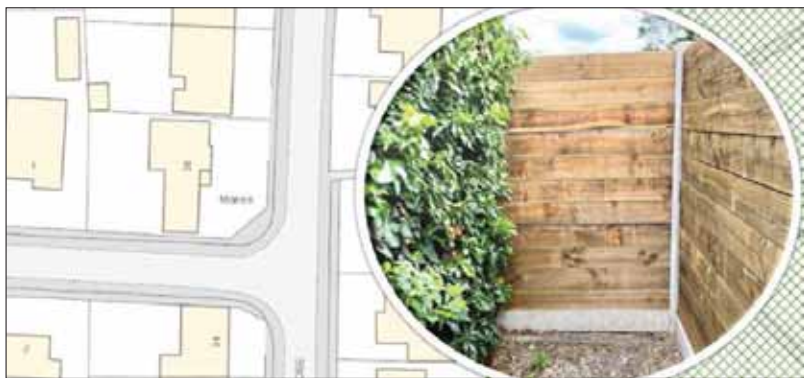
The fence closing off the footpath
