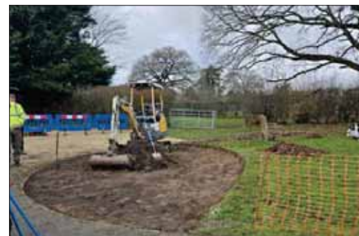
Works are currently under way for the new memorial
